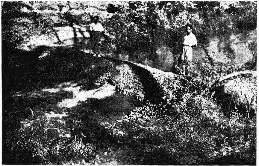
Figure 52. A small earth dam with oil-drum culvert outlet and hand-operated wooden gate, for stream flushing
